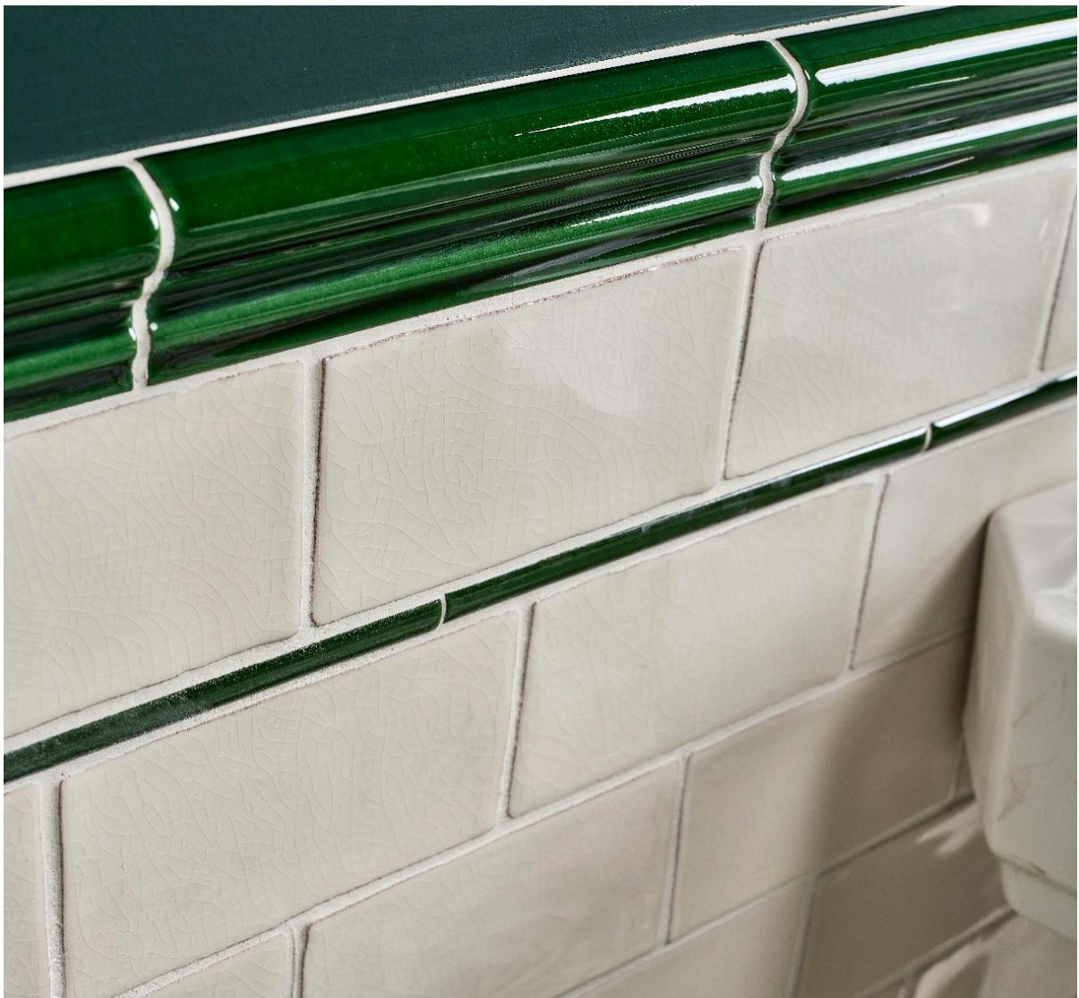
Crackle glazes are created when thicker tile glazes expand during the firing, then shrink when they cool. This causes the glaze to break in places, creating many tiny cracks. These cracks are very small and cannot be felt by touching- instead they appear as a lattice within the glaze of the tile.
