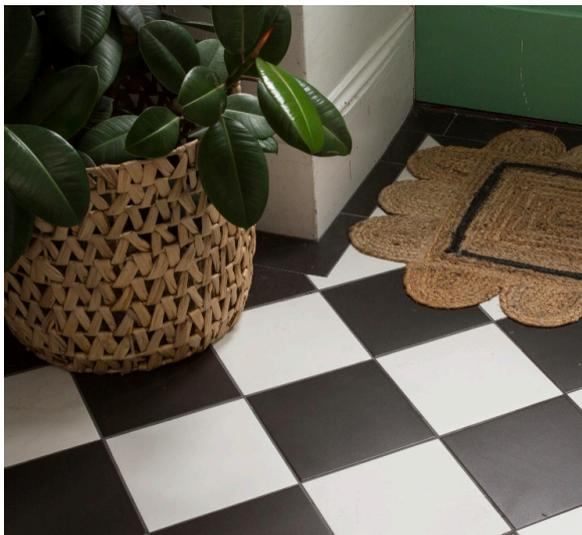
Generally, the tiles can be laid with wider grout joints than would be used for rectified products- this will absorb any difference in size.
